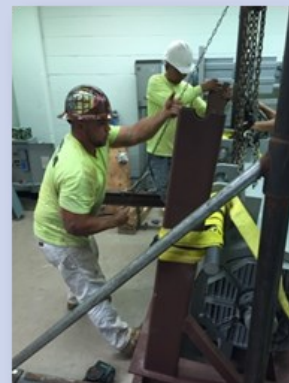
Equipment Relocation JBPHH
